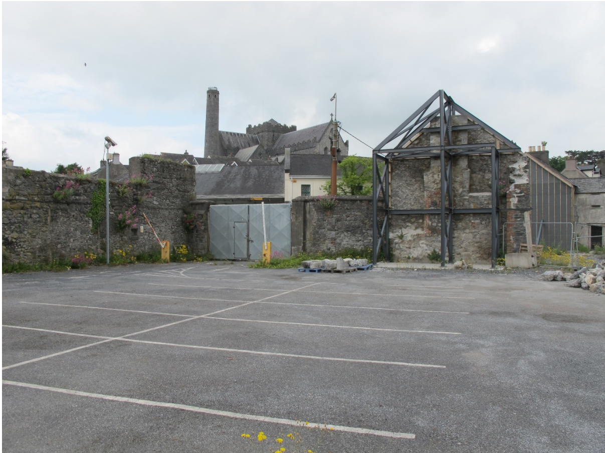
Plate 23: Braced gable of medieval to Early Modern house on 22 Vicar Street
