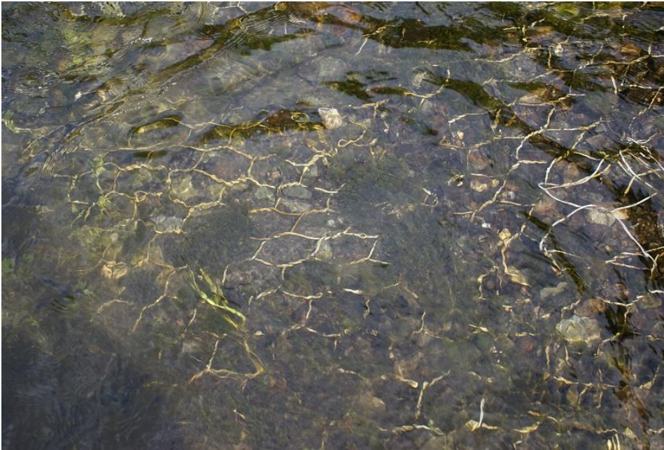
Photo 3: Gabion mattresses on bed of Breagagh River
