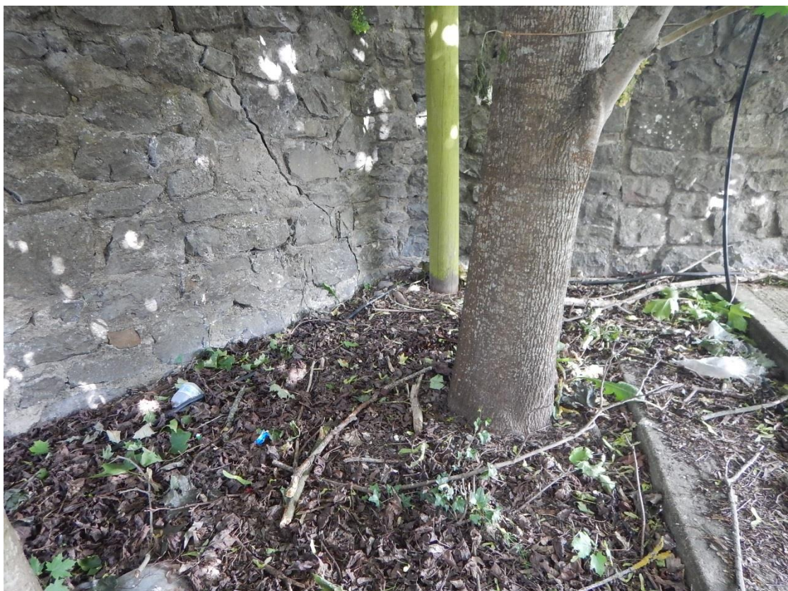
6. Crack in wall close to the base of tree T12
