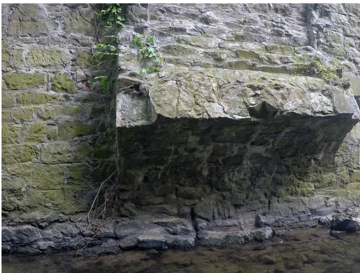
Plate 14 Springing for the south side of Cotteral's bridge (AMS 2018)
