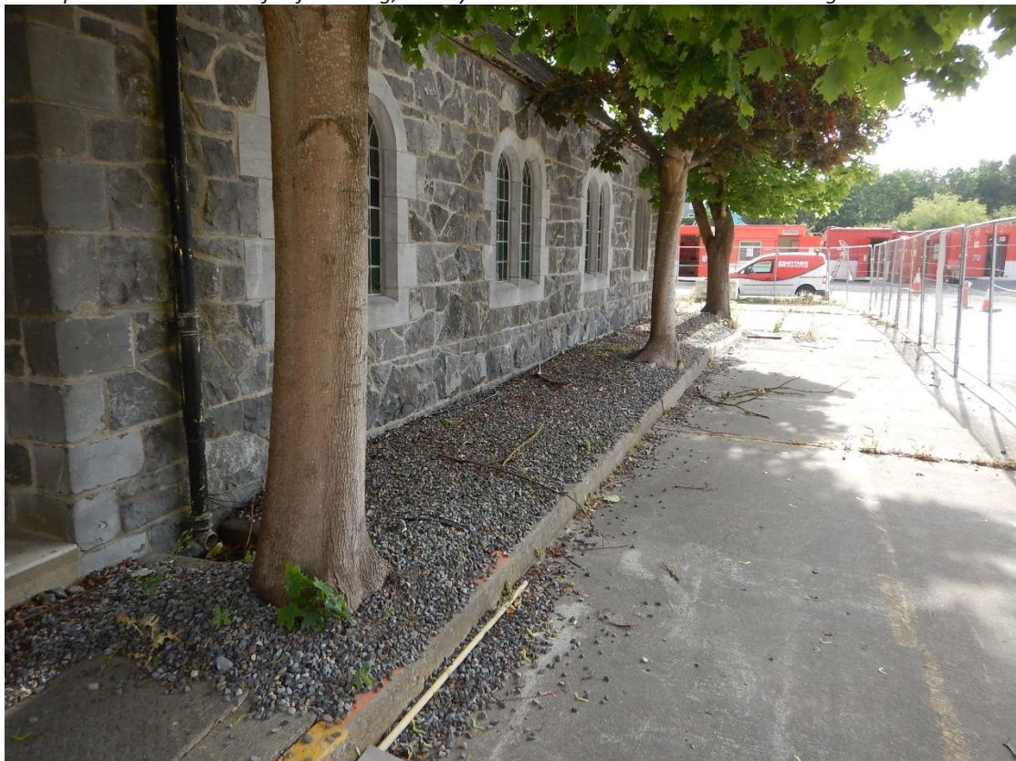
2. Trees T1-T3 showing close proximity of tree stems to building and very narrow verge in which the trees have been planted
